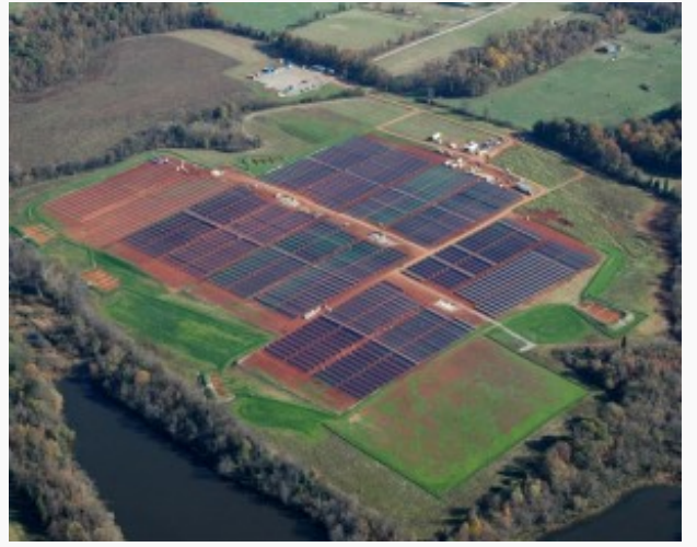
16-MW solar farm; Davidson County, NC
